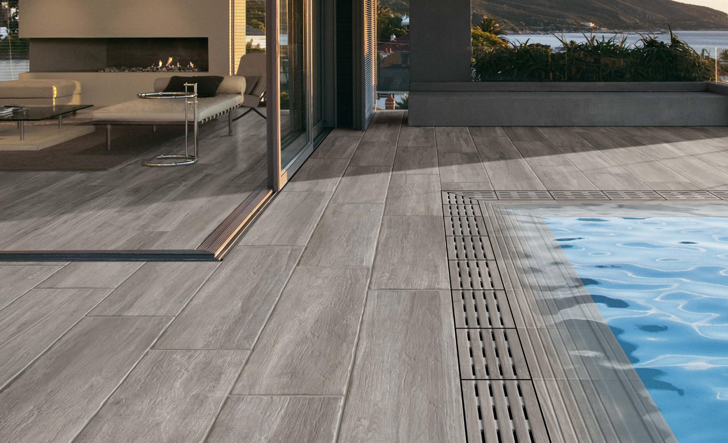
In order to get the overflow effect, one filter channel should be installed in all the perimeter of the pool, where water will be constantly flowing. This channel will be covered with our ceramic tile grill.
